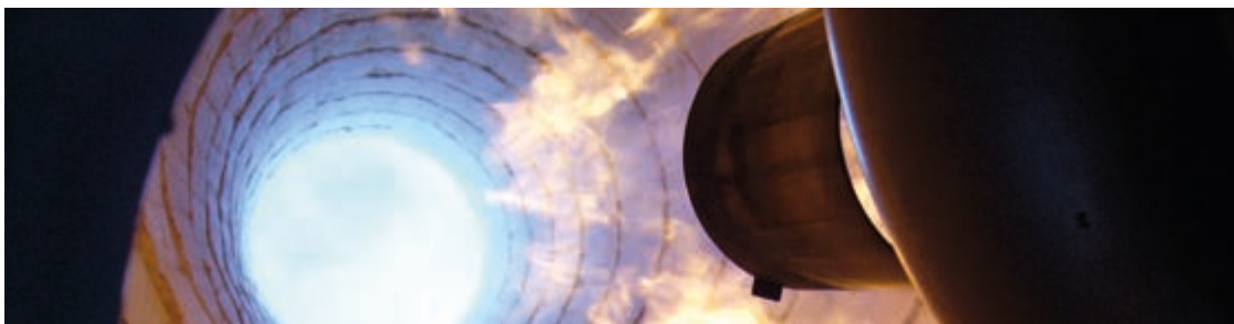
Inside a mobile combustion chamber – a flexible way to treat spent gas once a fermenter has been opened
